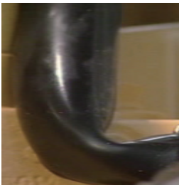
Air exhaust pipe is folded
